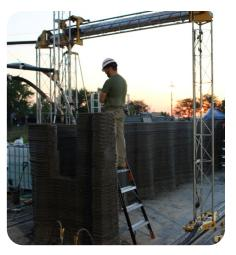
3D-Printed Concrete Barracks U.S. Army Corps of Engineers
