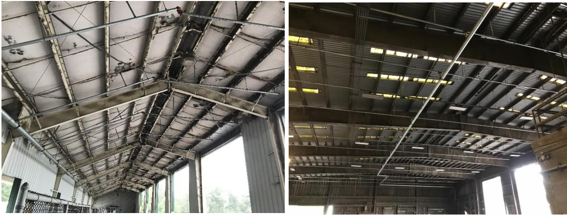
Figure 5.1: Existing Roof Structure
