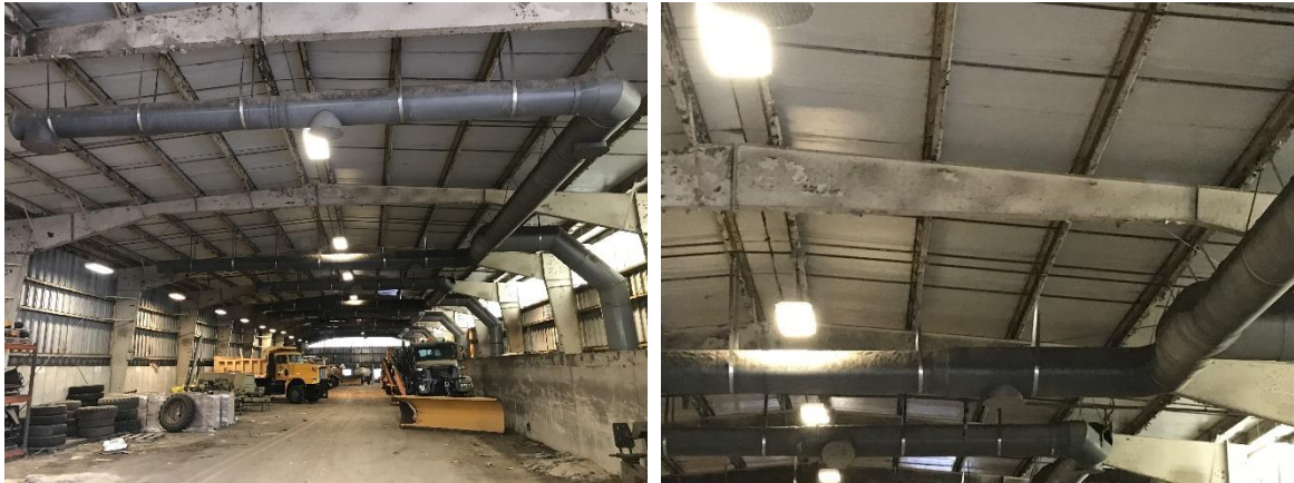
Figure 4.1: Existing Roof Structure
