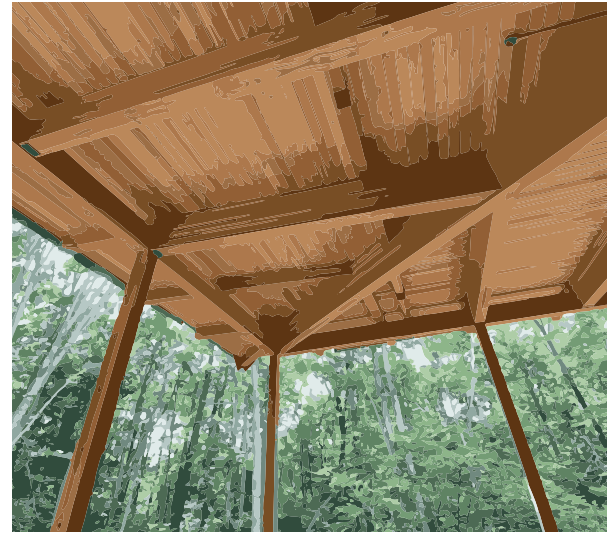
Norwell Public Library Glulam connection detailing
