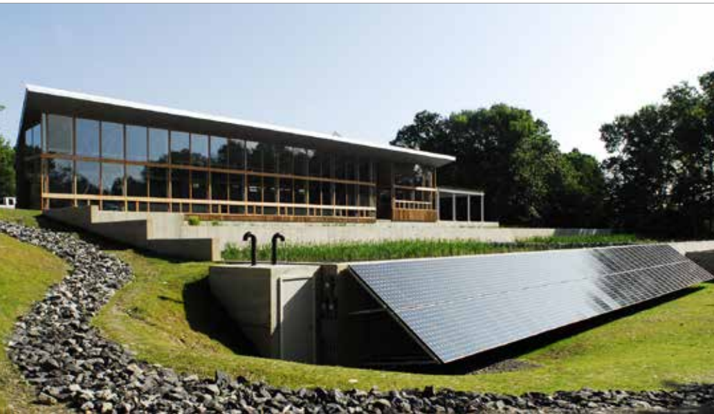
Left: Completed in 2009, the Omega Center for Sustainable Living is LEED Platinum and a certified Living Building.
