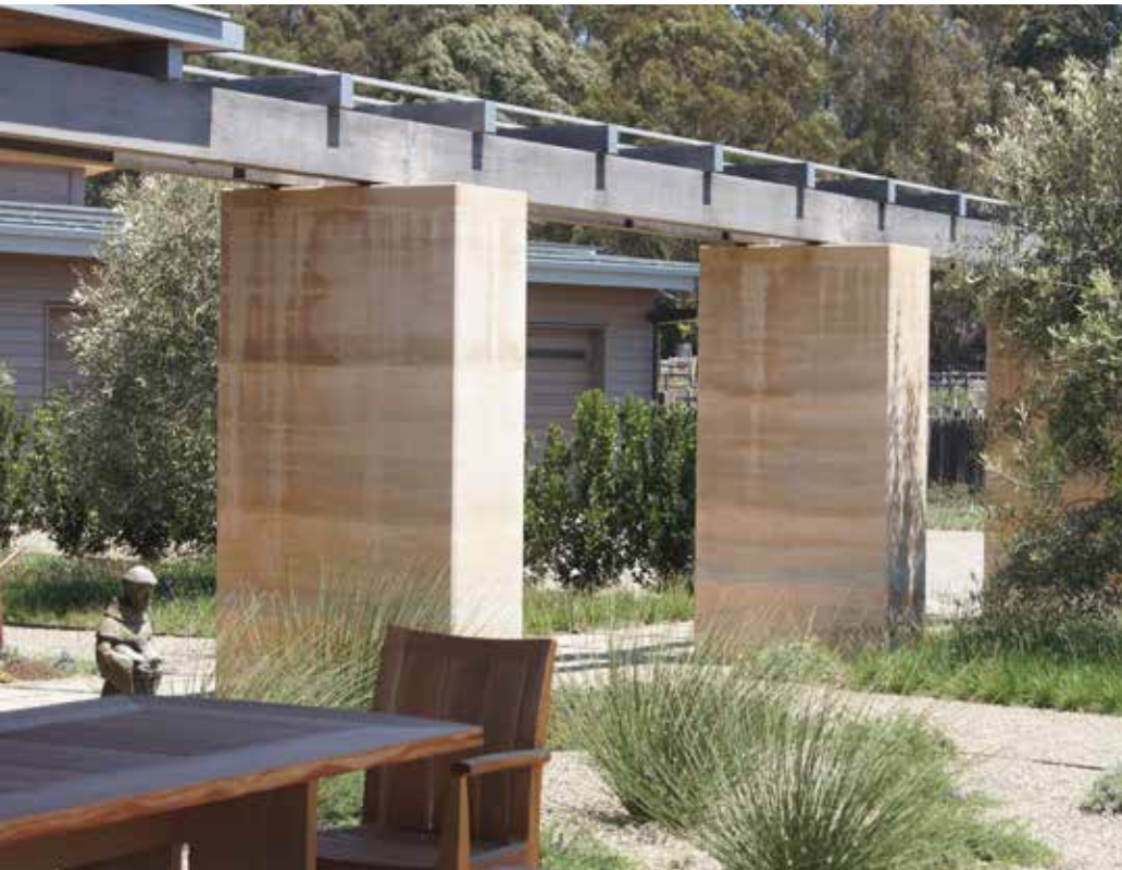
Left: Rammed-earth columns are used to meet the design goals of the architect and the client.
