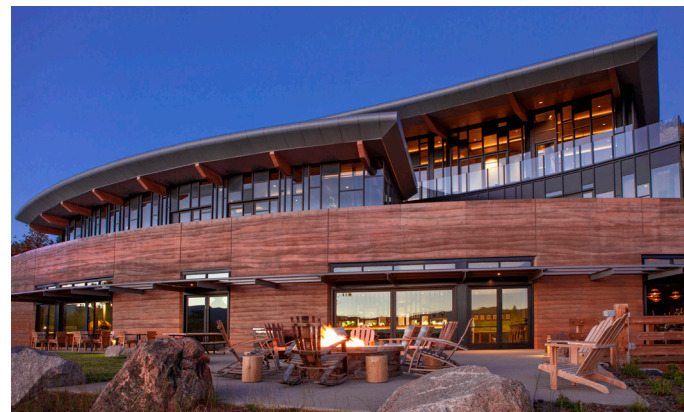
Lone Rock Retreat in Colorado utilized CLT and rammed earth walls. Watch a video.
