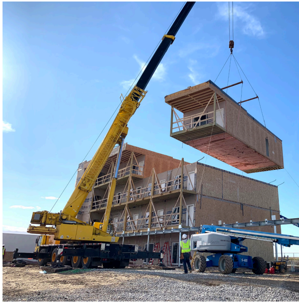
The Bend in East Moline, IL, utilized modular construction.
