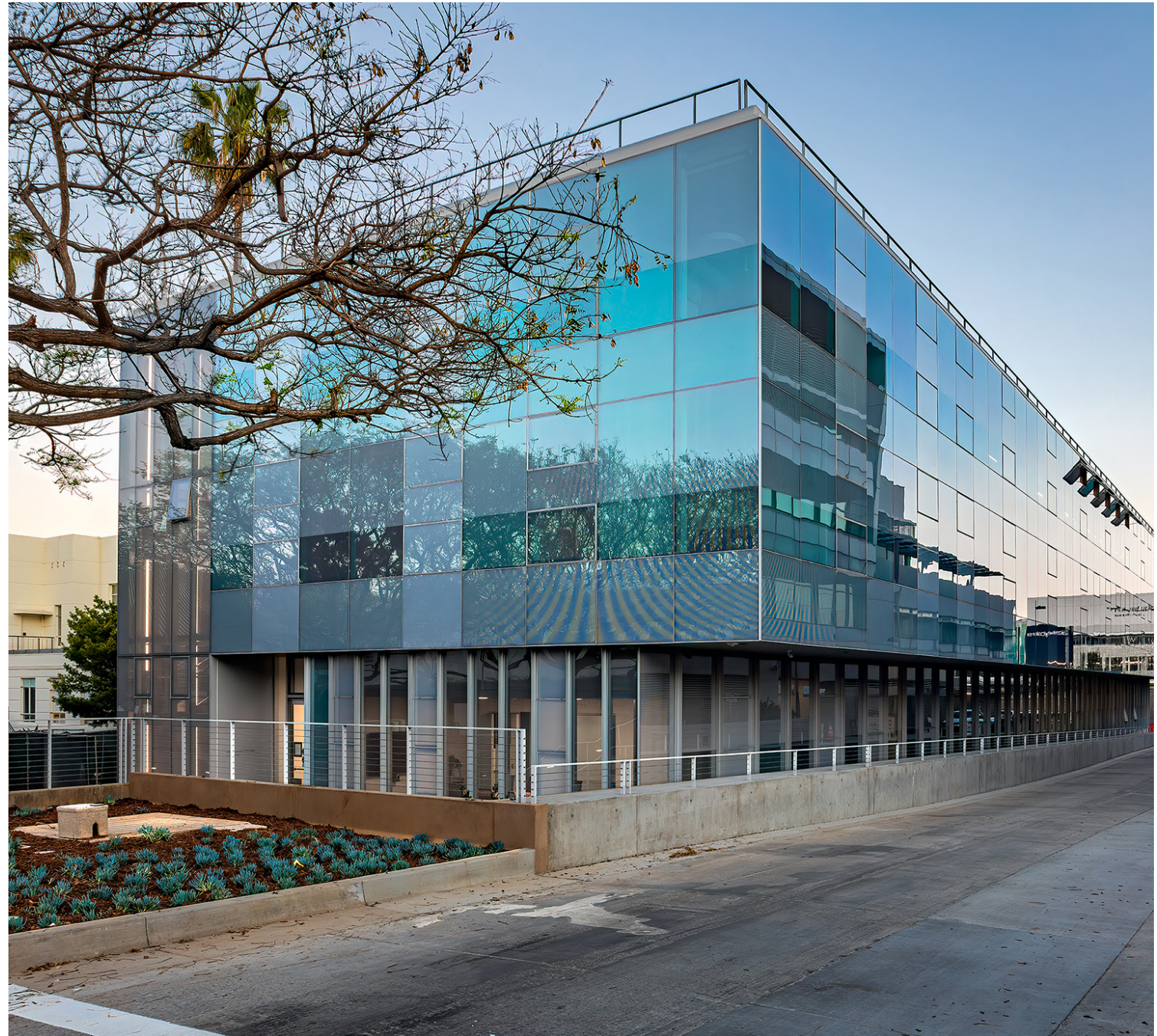
City of Santa Monica, City Hall East, Living Building Challenge Certified, Net Zero Water & Energy
