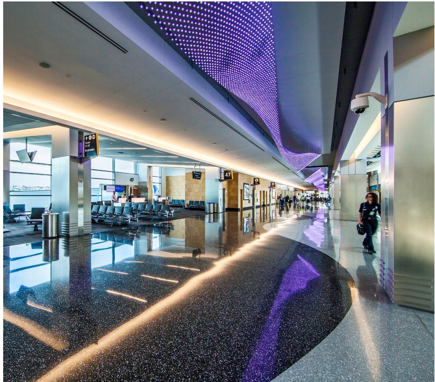
San Diego International Airport Airside Expansion, LEED Platinum (First airport project to ever achieve this goal)
