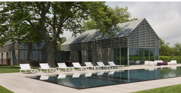
Above: Private residence structural engineering design and construction
