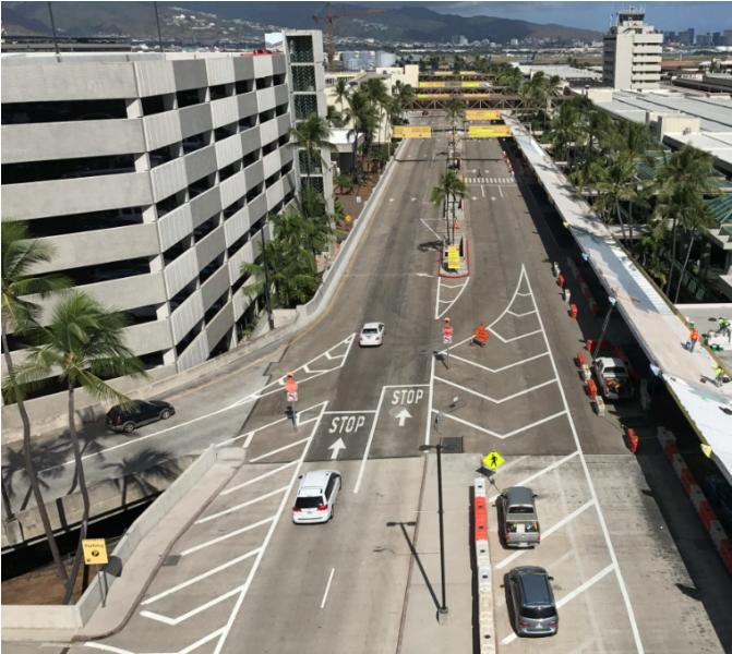
Daniel K. Inouye Int'l Airport Roadway Improvements
