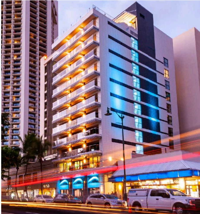
ESPACIO The Jewel of Waikiki Hotel - adaptive reuse
