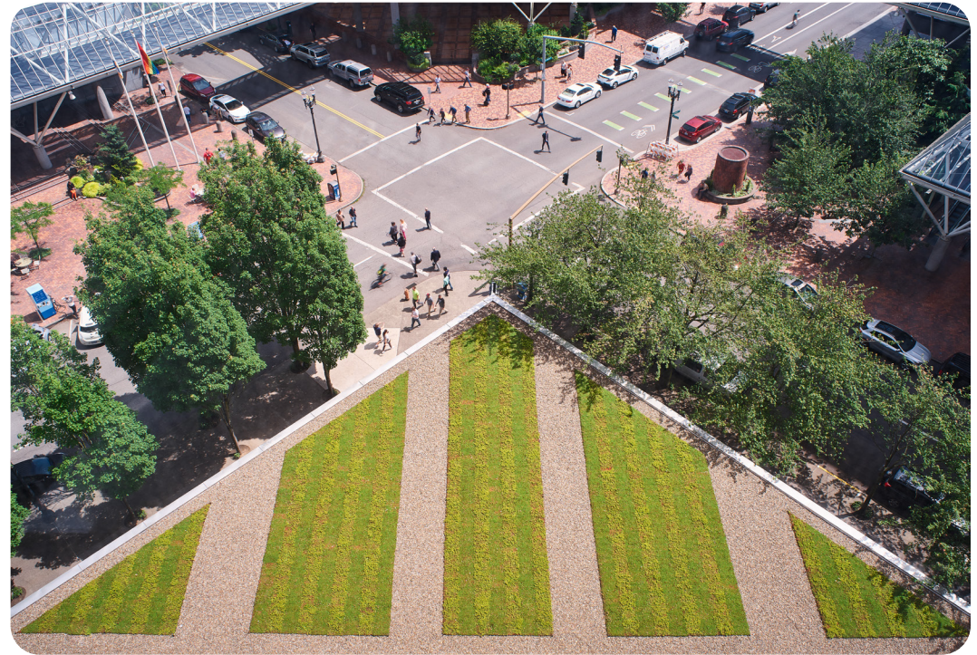
The design for One Main Place in Portland, OR utilized green roof to reduce water runoff and the heat island effects.
