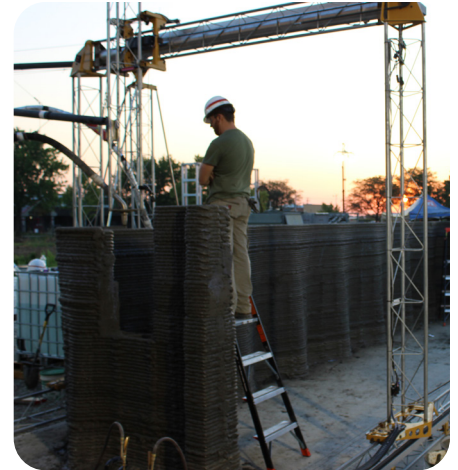
3D-Printed Concrete Barracks U.S. Army Corps of Engineers
