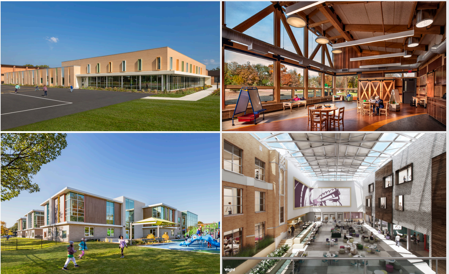
Images above: top left: Rhodes Elementary Classroom Addition, top right: Knoch Knolls Nature Center, bottom left: Lincoln Elementary School, bottom right: Downers Grove North High School Commons Roof
