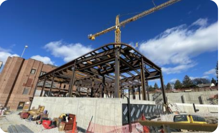
At Wellspring Health Surgical and Critical Care Tower, the concrete mix designs utilized type 1L cement, and steel column sizes were reduced through the use of 65ksi steel.
