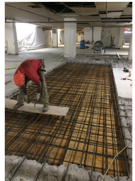
Below: Replacing the concrete slab on an existing parking deck.
