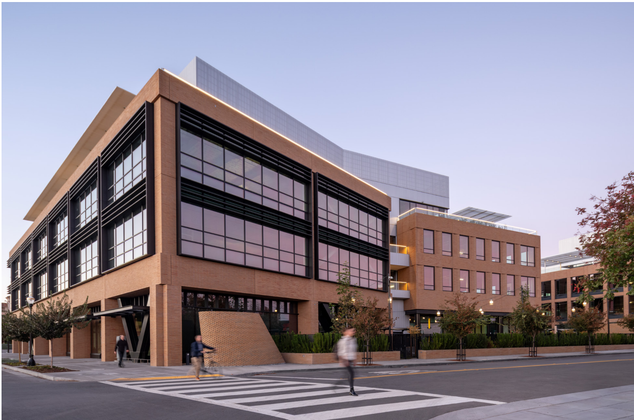
Elco Yards mixed use redevelopment, Redwood City, CA
