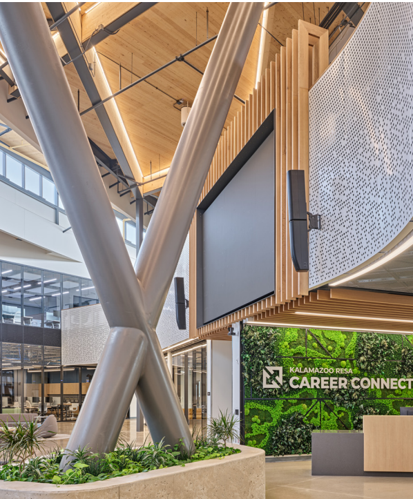
The KRESA Career & Technical Education Center in Kalamazoo, MI, features a hybrid steel-CLT structural system.
