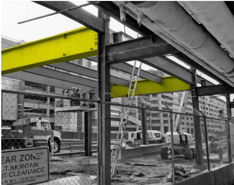
▲ Salvaged steel beams incorporated
